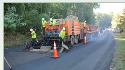
Typical micro-surfacing operation
